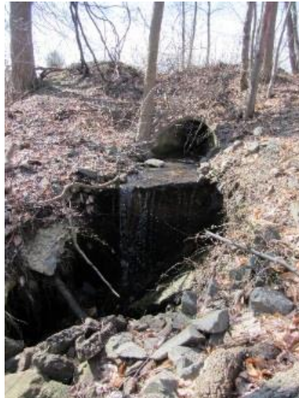
Outlet Destabilization
