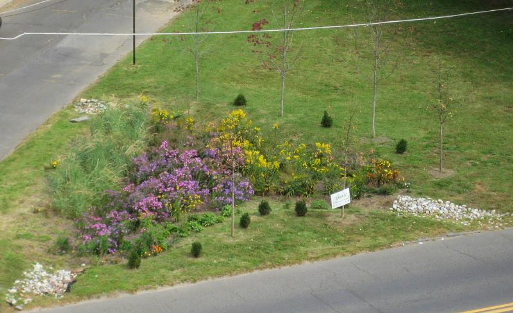
Bioretention Systems
