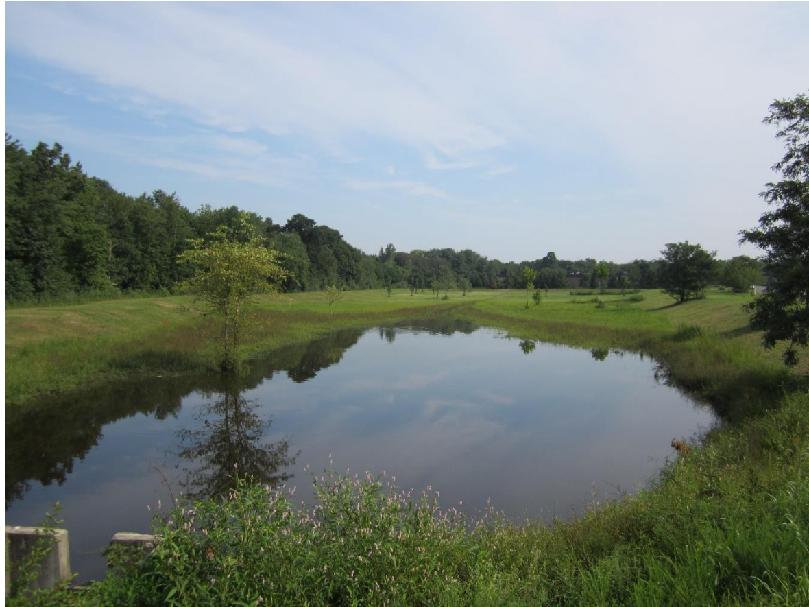
Standing water in detention basin
